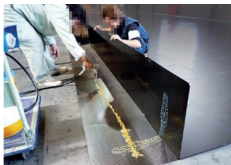
Application of Grease Seal
