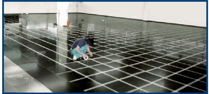
2 Install Sliding Plates
