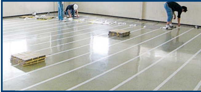
1 Install Cell Sheets
