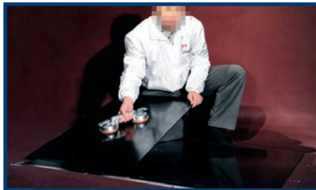
2 Install Base Steel Plate
