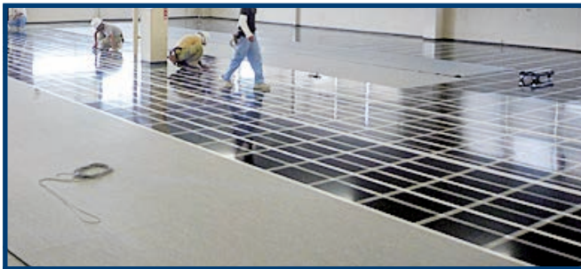
3 Lay Floor Covering
